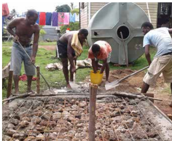
Men of Navakasiga help PCDF Engineers in the construction of the base for the first flush system water tanks.
