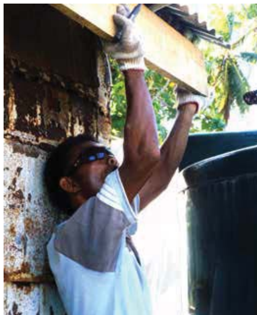
Akilio the hiring contractor replaces the facial board of a house in Batiki
