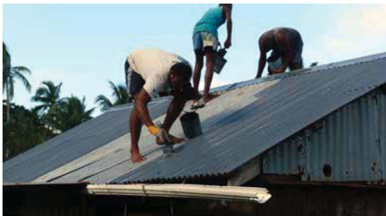
Communities help paint the roof as minor upgrades done to their rainwater system.
